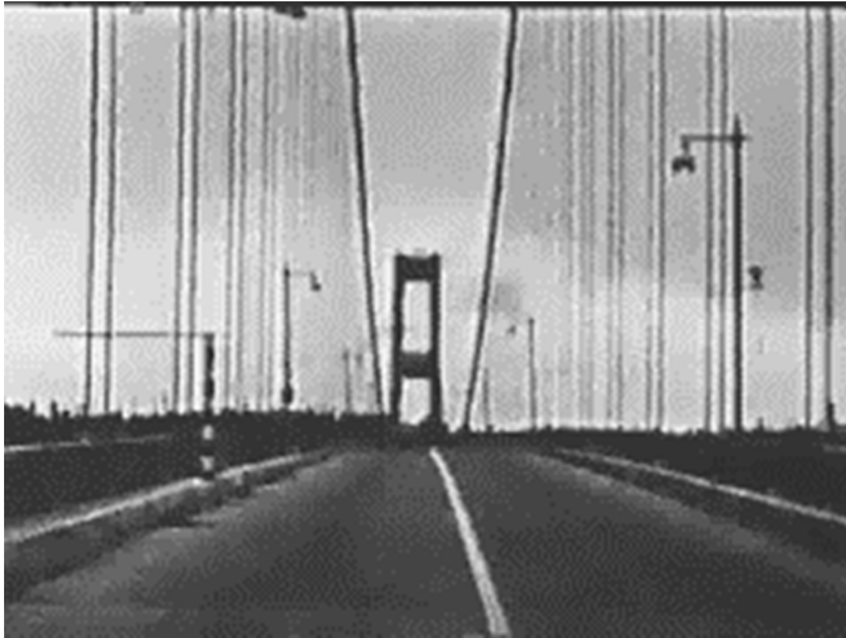
1st Juli 1940, Tacoma Narrows Bridge, USA
